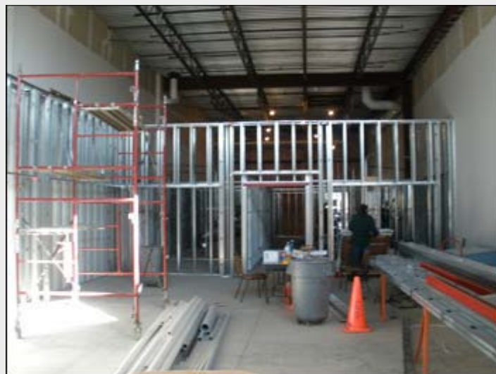
During Construction View
