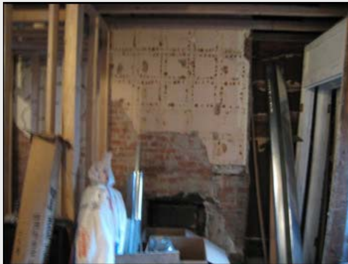
During Construction View
