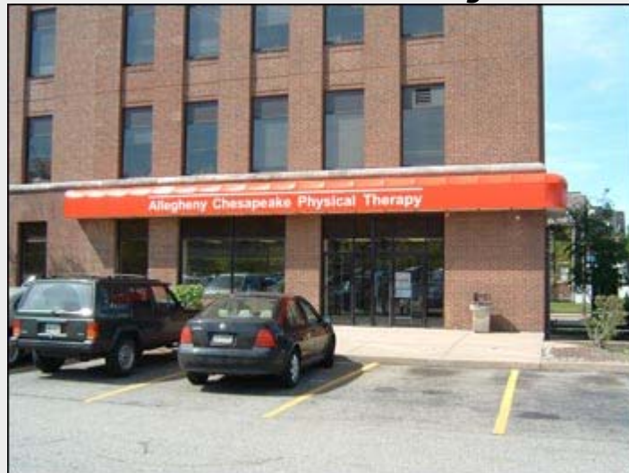
Exterior view of building
