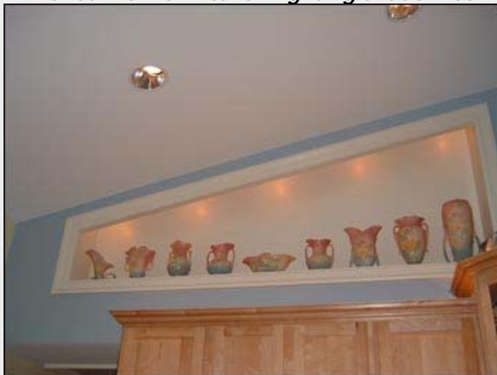
Finished view of kitchen lighting shadow box
