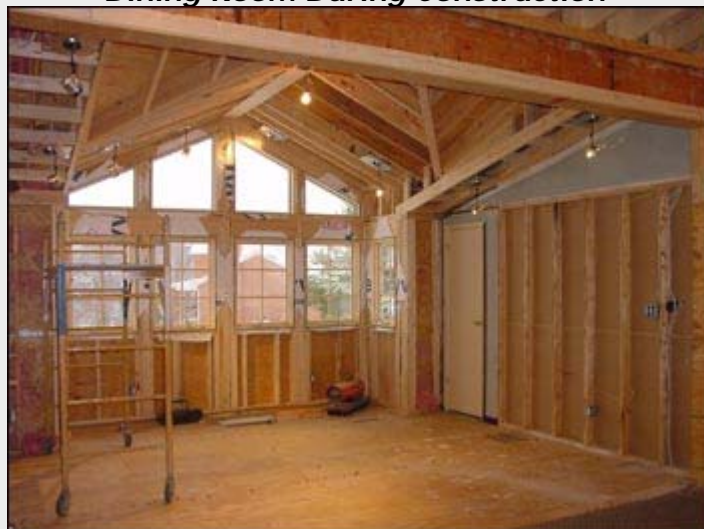
Dining Room During Construction
