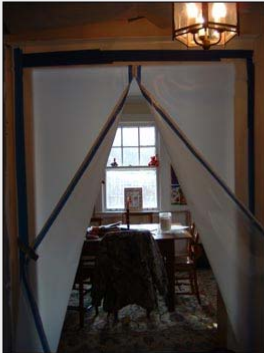
Zip Walls to keep dust out
