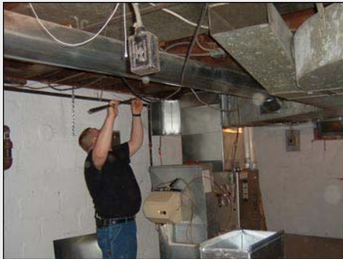
Ductwork Rerouting
