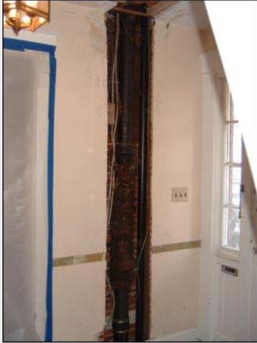
Sewer stack repair (notice how neat & clean)
