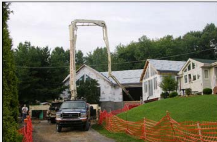
During Construction View
